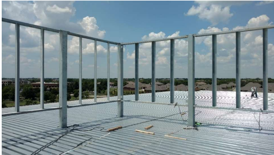
Figure 1: An Example of a Rooftop Screen Wall
